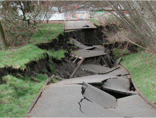
Lateral spread across a path at Capitol Lake, Olympia. Photo by Karl Wegmann (DNR)
