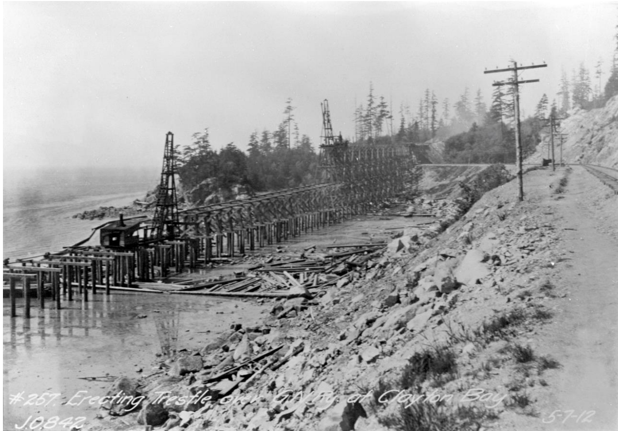
Figure 2. Clayton Beach 1912 Trolley Trestle Construction. Photograph taken from the south, looking north. Photo from Western Washington University Heritage Resources Archive.
