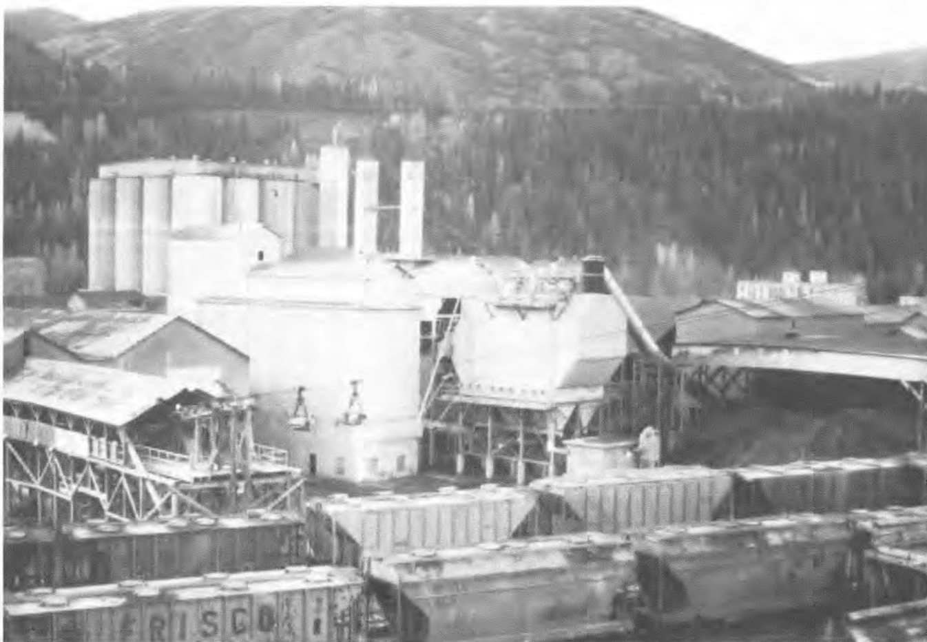
Portland cement plant in Metaline Falls purchased by Lafarge Corp. in 1989, showing aerial tram that transports limestone from the quarry.
