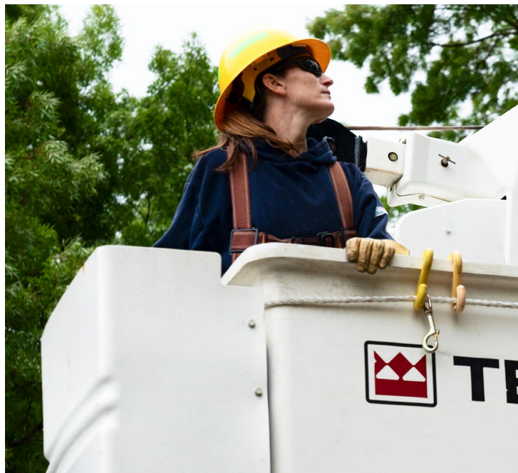
Crew conducting inspection/vegetation clearance around power lines.
