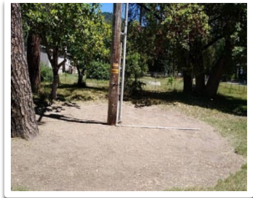
Figure 36: Pole Clearing at Pole Base
