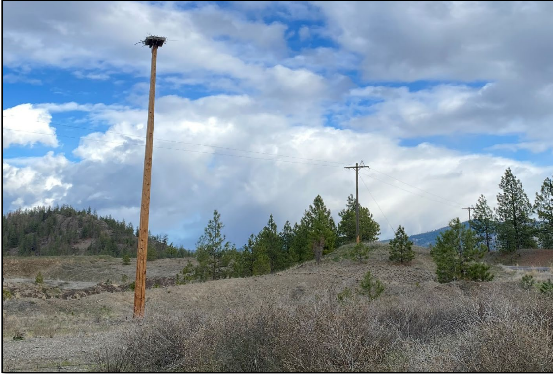
Figure 5. Nesting Platform and Perch Deterrent
