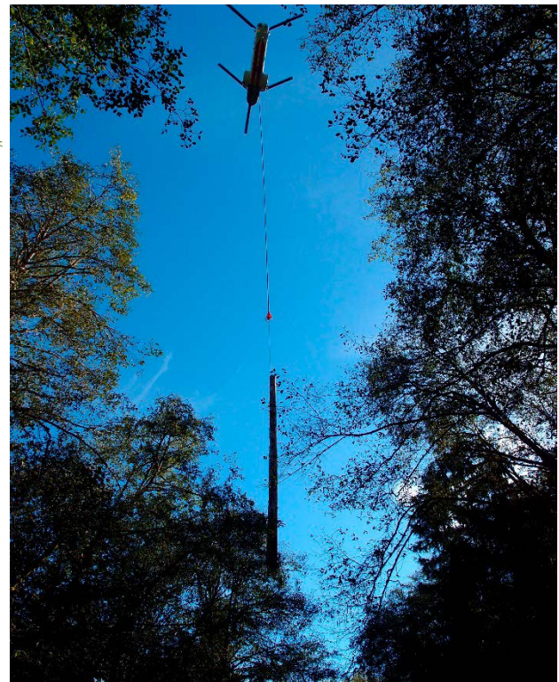
Photo 1. A helicopter prepares to place another log in Deep Creek during a logjam installation in 2012
