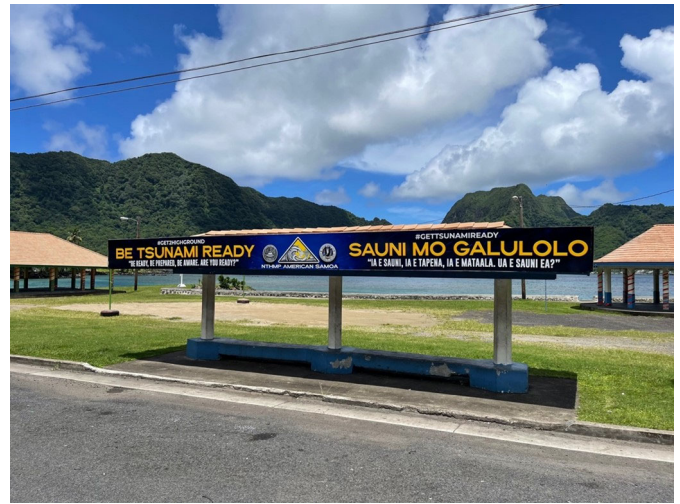
Bus stop in Utulei, American Samoa. Following the 2009 tsunami, the government procured and distributed Public Alert-certified weather radios to provide instant alerting to homes, schools, and businesses. Photo credit: Bruce Jones
