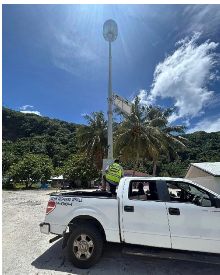
Siren maintenance and repair on Ta’u Island
