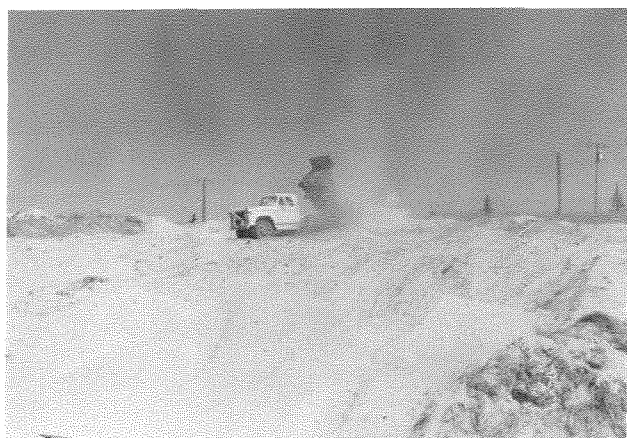
Figure 25.—Ash stockpile at Ritzville, Washington. Abandoned basalt quarry containing 103,000 cubic yards of ash.
