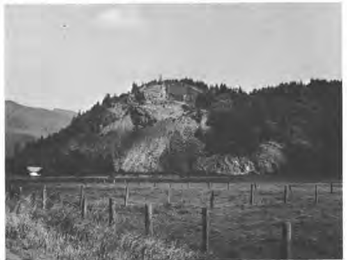
FIGURE 74.—Veazey quarry, near Enumclaw, King County, Washington. Columns and jointing, which are evident in the right and upper parts of quarry, control the upper limit of rock size that can be produced from the quarry.
