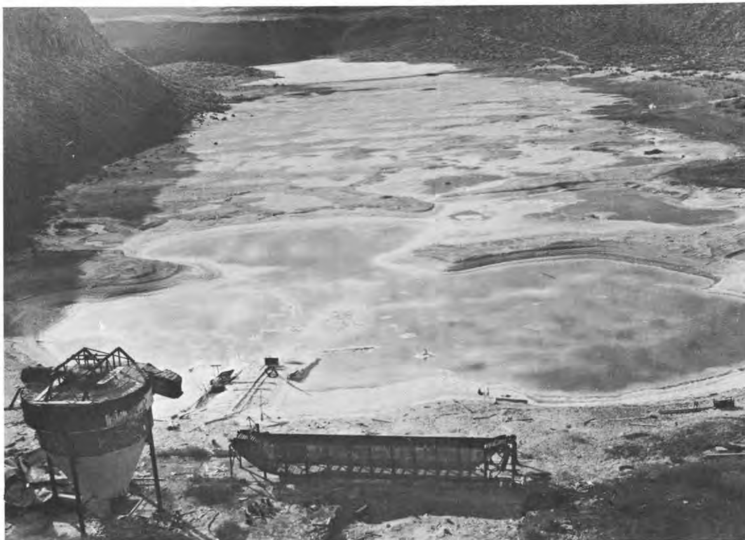
Figure 7.—Carbonate Lake. Note the mottled appearance of the salt bed in the brine pool in the foreground at the north end of the basin, irregular salt crusts surrounded by gray, fluffy mud areas in the center of the basin, and a vat of salts from evaporated brine at the extreme south end. An old evaporator (left) and settling tank stand in the foreground. October 1945.
