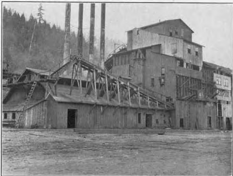
B. Boiler House and Washer, Wilkeson Coal & Coke Company.
