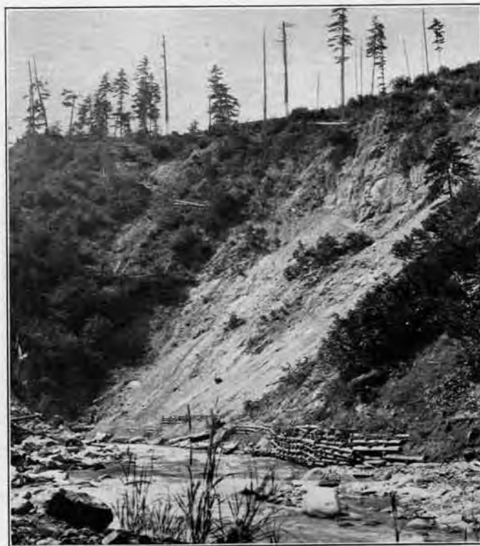
B. Carbon Canyon Looking Downstream From South IX Tunnel.
