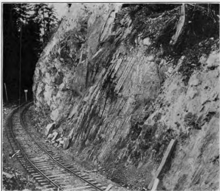
A. Contact of Andesite Dike and Shales Near Fairfax.
