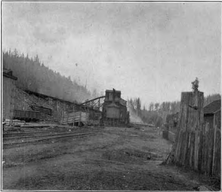
A. General View of Washer and Ovens. Wilkeson.
