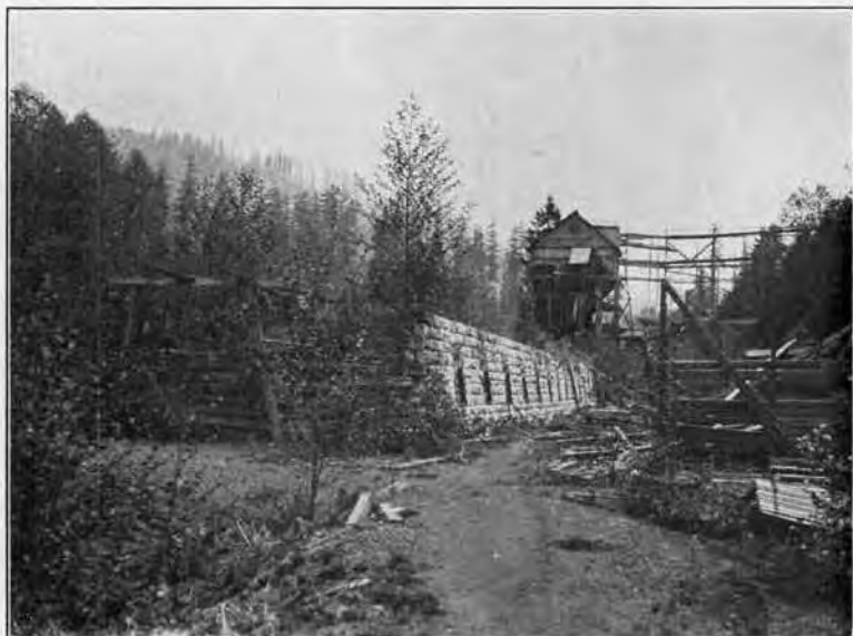
B. Coke Oven Plant at Montezuma.
