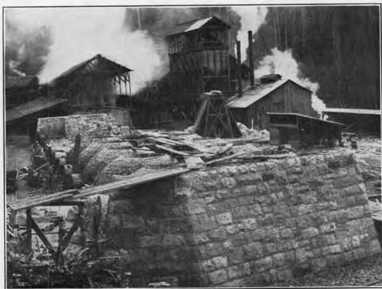
B. Carbonado. Coke Ovens and Coal Bins.
