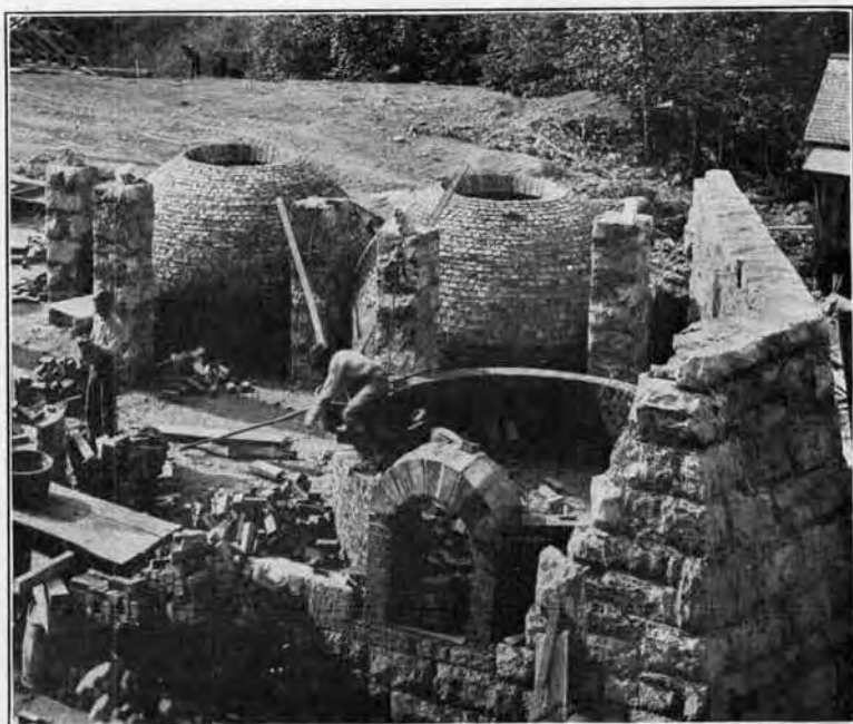
A. Carbonado. Coke Ovens Under Construction.
