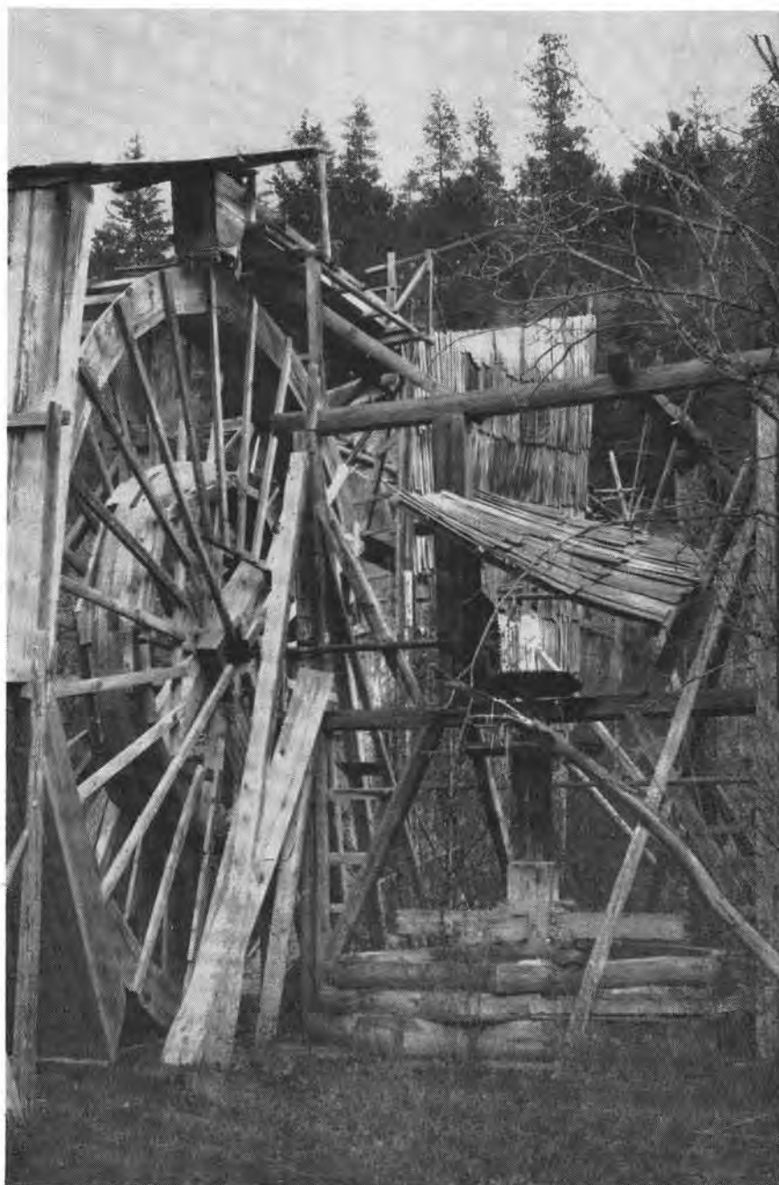
OLD ARRASTRE AT LIBERTY, KITTITAS COUNTY, AS IT APPEARED IN 1924 Powered by overshot water wheel
