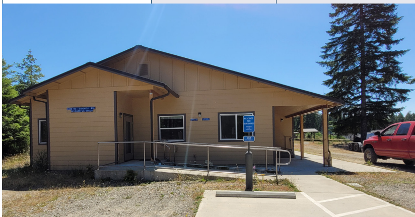
Building SP0210—Belfair Work Center. Constructed during the 19-21 Biennium with capital funds, the building was completed in the spring of 2021. The building is approximately 3100 sq.ft. in size and replaced a mobile office trailer that had been in place as a DNR office for nearly 30 years. The building accommodates roughly 18 personnel depending on configuration and use pattern. The project cost roughly $1.5 Million and utilized a pre-manufactured construction method.
