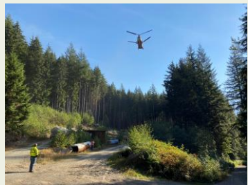
Helicopter bridge installation
