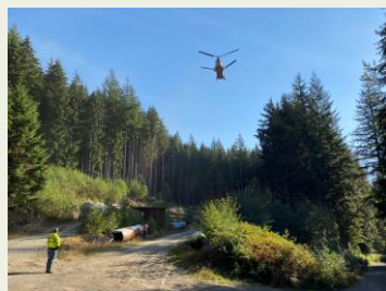
Helicopter bridge installation
