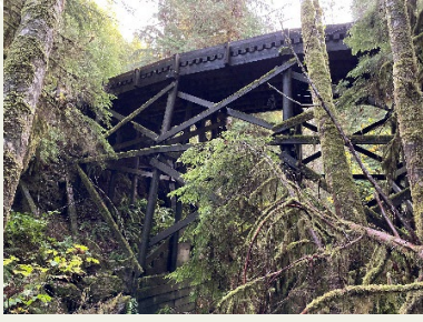
Kostly Creek Bridge
