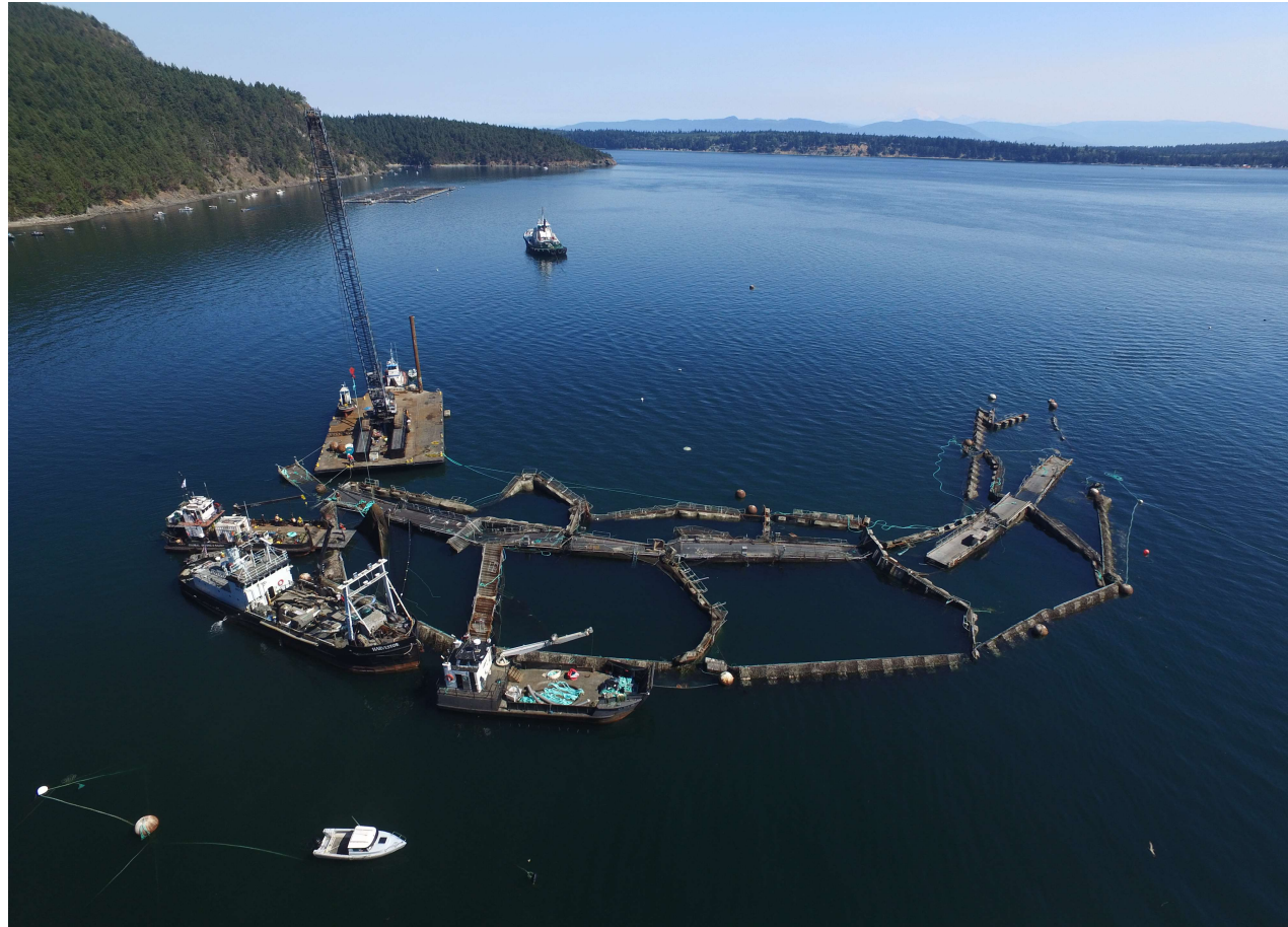
DNR drone image of collapsed Cypress Island net pen #2 in Deepwater Bay, August 28, 2017.
