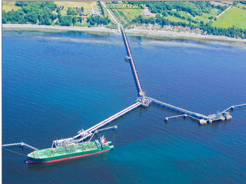
Figure 18. bp Pier ( Ecology Coastal Atlas ).
