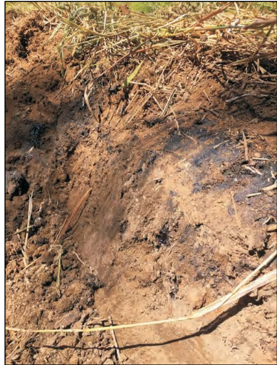
Figure 6. Oil pockets in soil from prolonged leaking under storage tanks. Photo taken by Valeriy Bizyayev, 7/31/17. EPA Assessment and Emergency Removal Final Trip Report (Nov. 2017).
