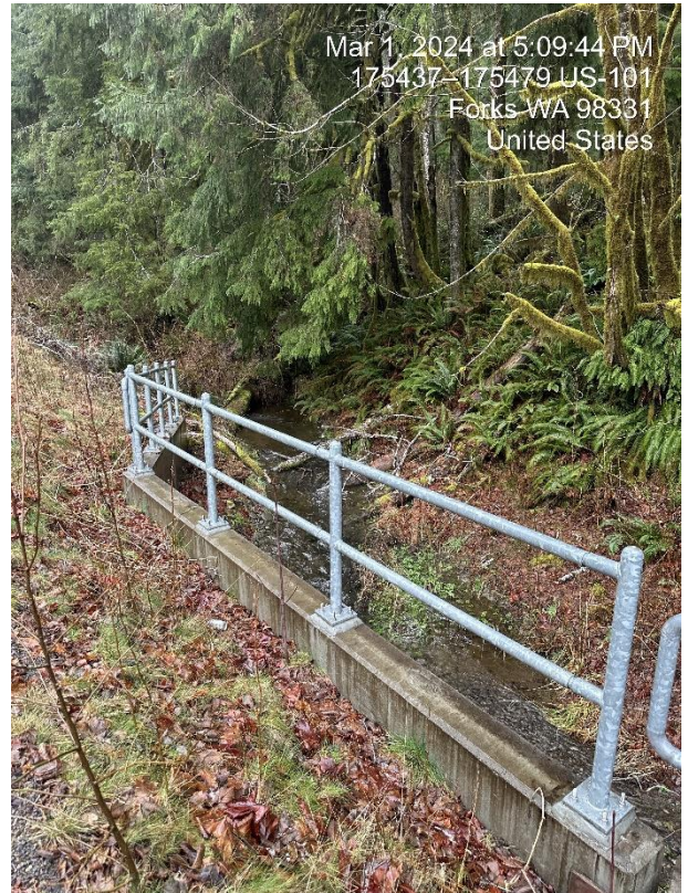
Image 9. Culvert at toe of slope near HWY 101
