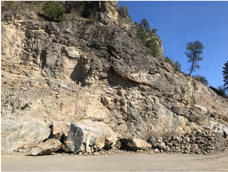
MINED EXCAVATION INTO CONGLOMERATE AT NAFF PIT. BEDDING DIPS DOWN AND TO THE RIGHT (SOUTHWEST). ROCKFALL HAS ACCUMULATED AT THE FOOT OF THE HIGHWALL. PHOTOGRAPH TAKEN FACING EAST.
