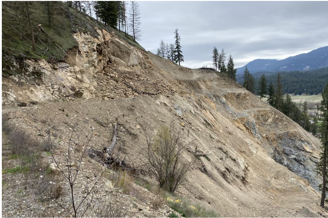
OVERSTEEPENED BENCH WALL AND ROCK DEBRIS IN CUT 2. OTHER BENCHES AND THE TALL SOUTH WALL OF CUT 1 ARE VISIBLE AT RIGHT. VIEW IS TO THE SOUTH.
