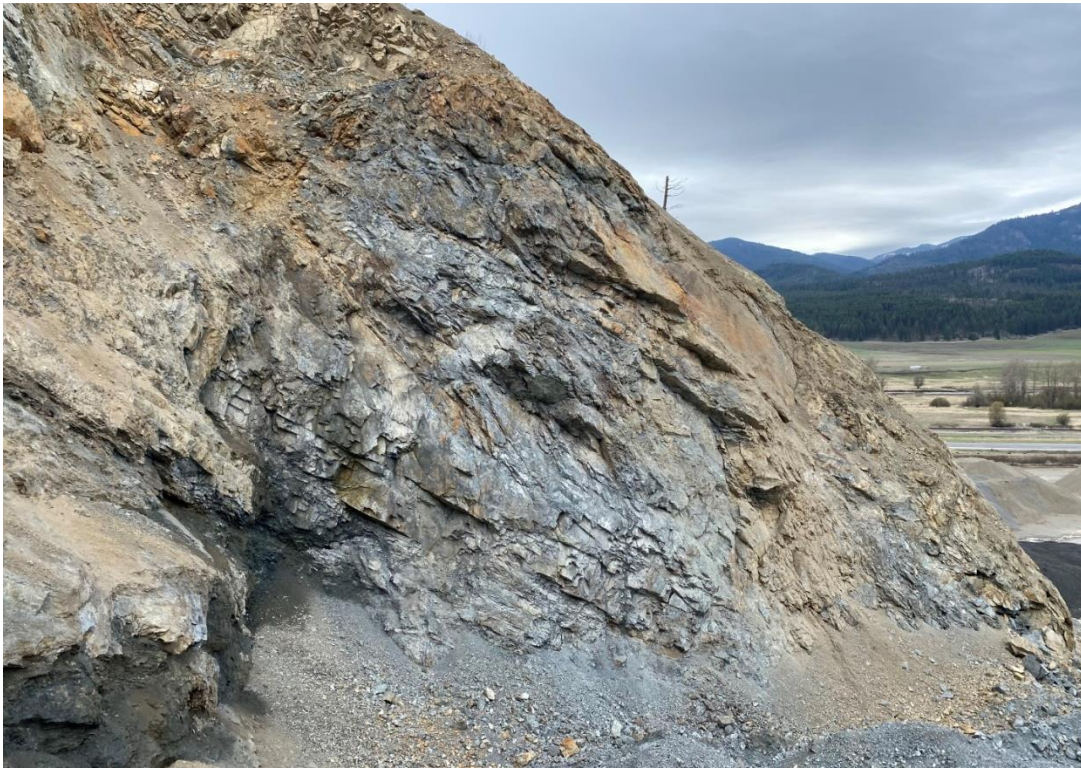
PROMINENT, SOUTHWEST-DIPPING BEDDING IN CONGLOMERATE EXPOSED IN THE SOUTH WALL OF CUT 1. VIEW IS TO THE SOUTH.
