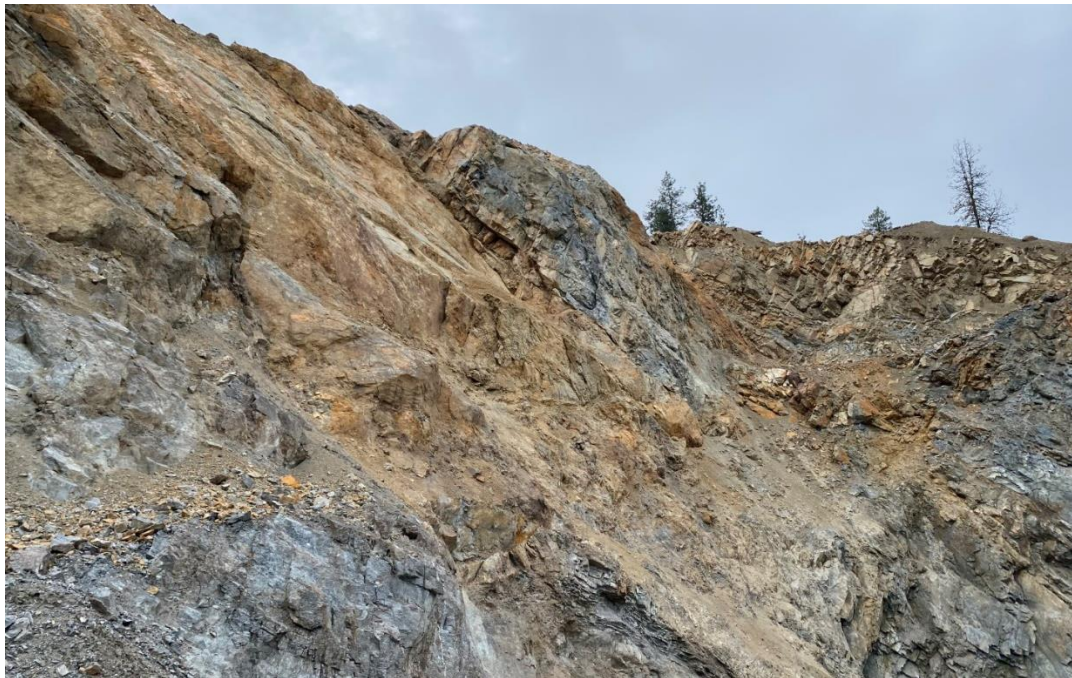
SUSPENDED BLOCK OF CONGLOMERATE (GRAY) IN CUT 1. NOTE THE ORANGE-STAINED, ANGLED BEDDING PLANE IN THE FOREGROUND LEFT OF THE BLOCK, WHICH LIKELY UNDERLIES THE BLOCK. VIEW IS TO THE SOUTHEAST.
