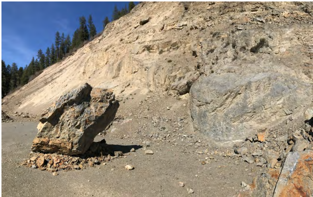
ROCKFALL BOULDER APPROXIMATELY 8 FEET IN DIAMETER. THE MINED SLOPE IN THE BACKGROUND IS MOSTLY FORMED FROM REMOVAL OF TALUS. PHOTOGRAPH TAKEN FACING NORTHEAST.
