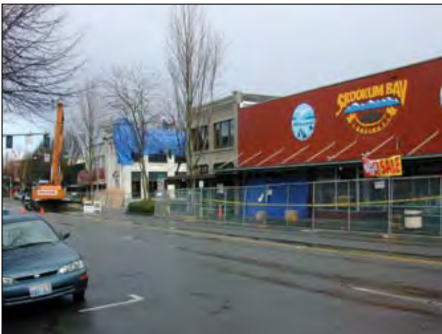
Closed businesses and disrupted streets, like this one after the Nisqually earthquake, can be a problem for the economic health of communities. Photo: Robert J. Reid
