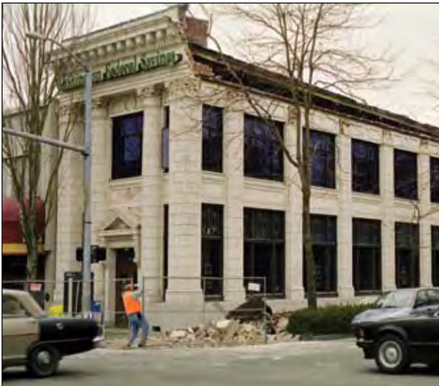
This photo of a building in Olympia after the 2001 Nisqually earthquake shows typical damage from a deep earthquake. A major source of injury is falling parapets, such as those seen above. Photo: Josh (Robert) Logan, DGER
