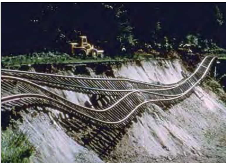
Landslides are an often-overlooked danger of earthquakes. They are particularly likely during rainy, water-soaked winter months in Cascadia. Almost 40 miles (60 kilometers) from the epicenter, this section of the Union Pacific Railway was left dangling after the hillside fill beneath it slid away in the 1965 earthquake. A sewer main also broke. Photo: University of California, Berkeley
