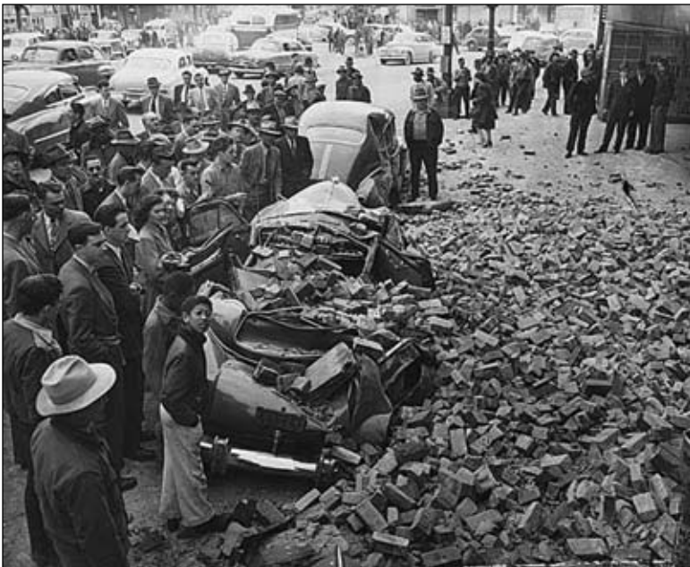
During the April 1949 earthquake, the owner of the Busy Bee Cafe barred the doors to keep panicking patrons from rushing outside. Seconds later, brick fell from the top of the Hotel Seattle, crushing several cars. Photo: Seattle Post-Intelligencer Collection, Museum of History & Industry; All Rights Reserved
