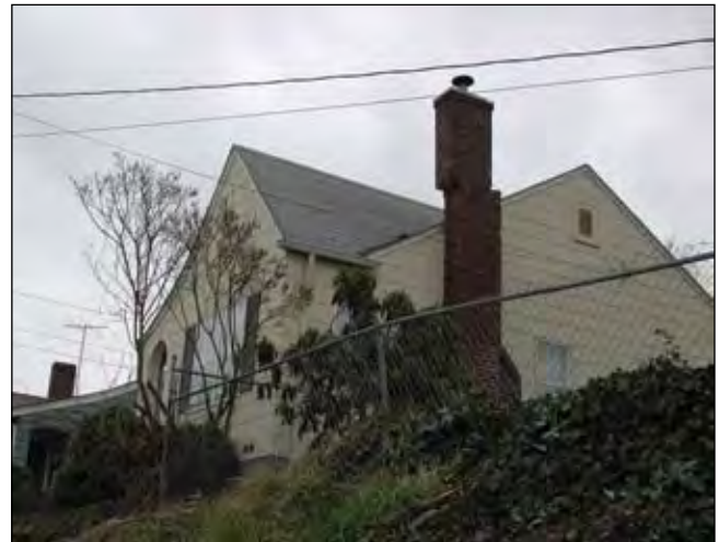
Chimney failures are a common problem for homeowners after an earthquake. The above chimney did not fall but remained a safety hazard until it was rebuilt. Photo: Michael Polenz, DGER
