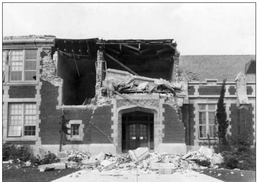
The Long Beach, California school above shows how dangerous old, brick buildings can be. In the 1949 Olympia earthquake, the Senior Class President of Castle Rock High School was killed by falling bricks. The gable on the school collapsed, even though the structure was more than 50 miles (80 kilometers) from the epicenter. Photo: USGS
