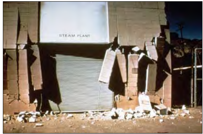
The 1971 San Fernando earthquake substantially damaged these Juvenile Hall facilities. A portion of the two-story administration building collapsed completely into the first story. Photo: E.V. Leyendecker, USGS
