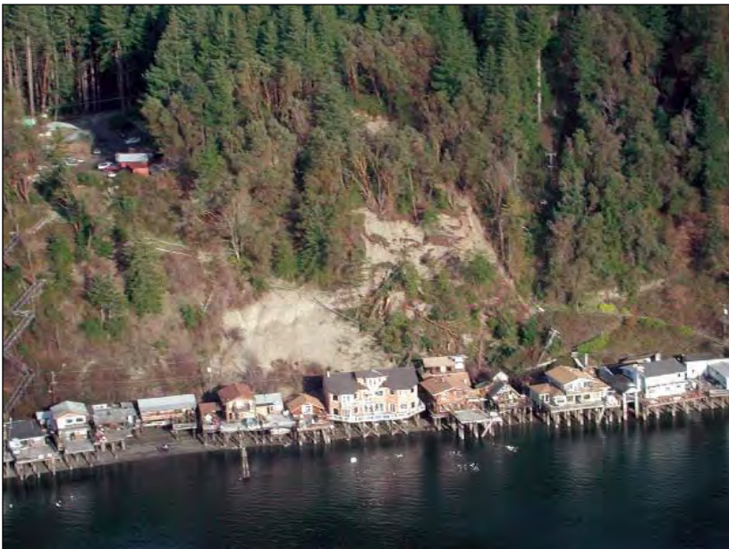
Salmon Beach, near Tacoma, was the site of a landslide three days after the 2001 earthquake. The same hillside slid after the 1949 event. Photo: Dave Sherrod, USGS
