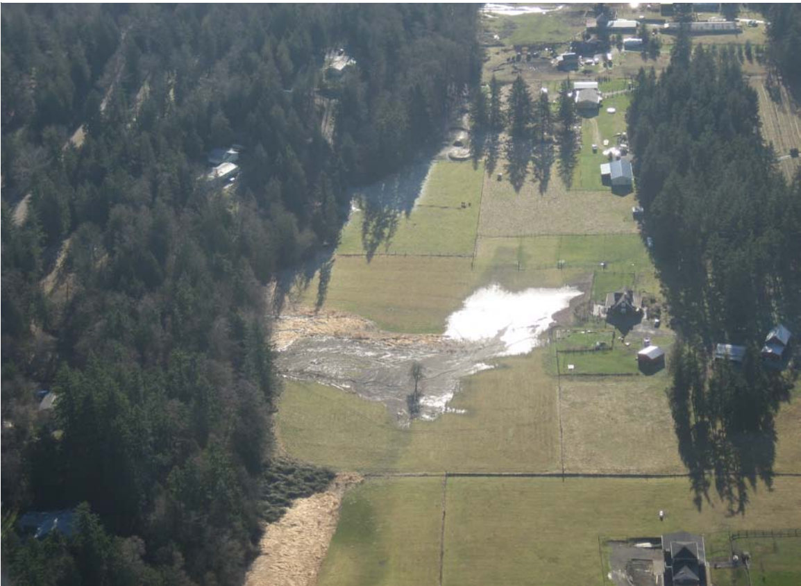
Figure 12 Aerial photograph of flooded area east of 6489 Siper Road. Residence is structure just to right of ponded water. View looking to south. Photograph take 1/20/09. (Photo by D. Hooks)
