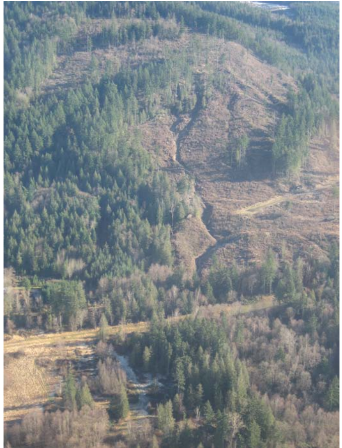
Figure 4 Aerial photograph showing debris-flow track (furrow on hillside) from PIs to pipeline right-of-way (grass strip across lower area of photograph). Treeless areas delineate Gasping Goodwin Aerial timber sale. View looking southeasterly. (Photo by D. Hooks)
