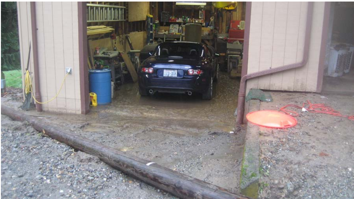
Figure 10 View of garage at 6489 Goodwin Road and pole placed to divert debris. Some debris entered garage before placement of pole. View looking southwest at southeast corner area of garage. Photograph taken 1/8/09. (Photo by D. Hooks)
