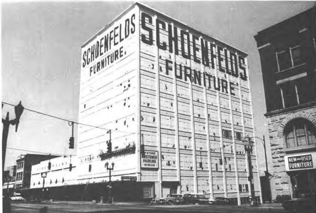
Figure 23.—Glass windows broke on three sides of this 10 story building in Tacoma. The fourth side had no wall openings. (Photo by B. J. Morrill.)
