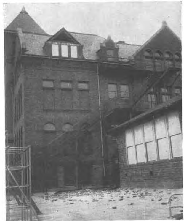
FIG. 8—School in Tacoma. The gable wall fell and killed a small boy.
