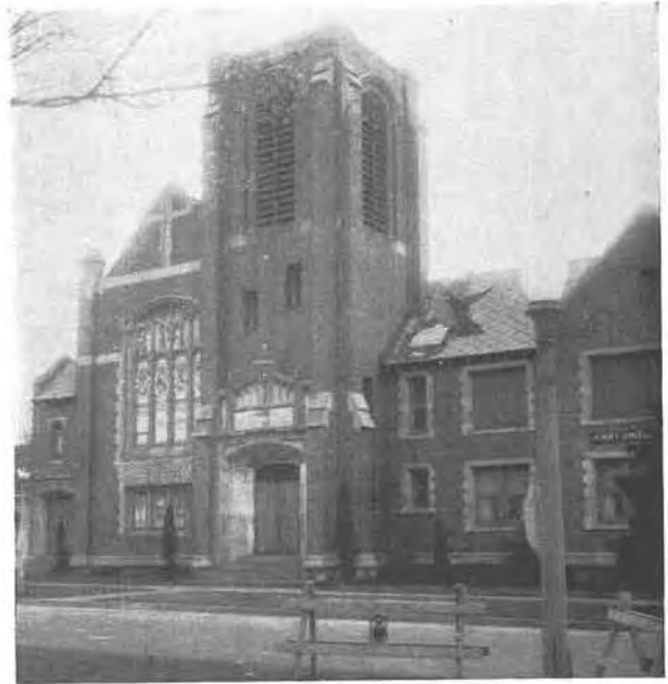
FIG. 7—This church steeple in Tacoma had a spire at each corner. The spires were thrown off and two of them went through the roof of the building.
