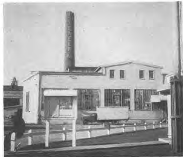
FIG. 14—Industrial plant at Olympia. Brick chimney was originally 250 feet high; about 60 feet of the top was thrown off, producing fatality.
