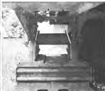
BRIDGES damaged by the quake. Left—Horizontal reinforced concrete struts between viaduct and trestle in Spokane were destroyed by differential movement of the structures. Below—Adna bridge over Chehalis River moved perpendicular to center line of road to bend pin plates on all shoes.
