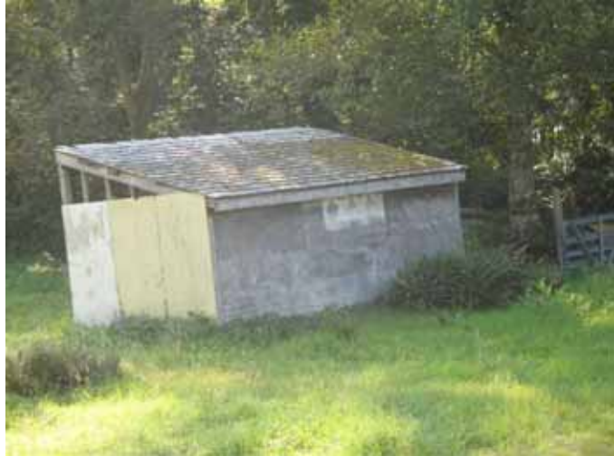
Figure 5-12: Outbuildings are often overlooked when mitigating wildfire risk.
