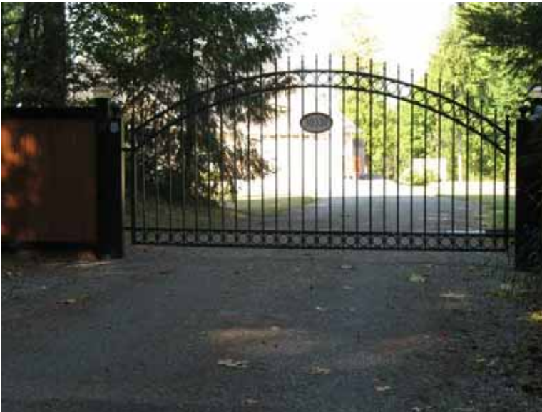
Figure 5-17: Locked gates can prevent responders from accessing a property during an emergency.
