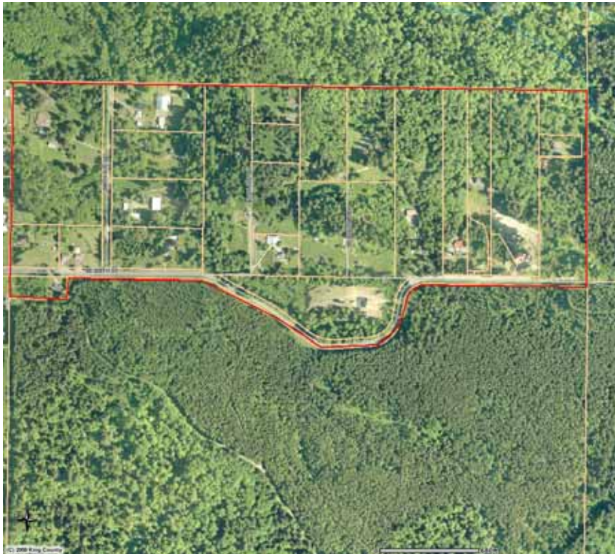
Figure 4-1: Northeast Hobart Firewise planning area boundaries in red with parcels shown in yellow. (King County GIS)
