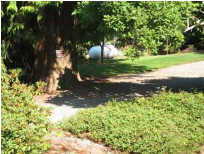
Figure 5-13: Above ground propane tank with nearby flammable materials.
