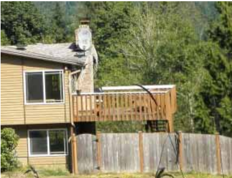
Figure 5-10: Wooden fences connected to a residence can spread fire to the home. In this case opening the gate would prevent fire from traveling to the main structure.
