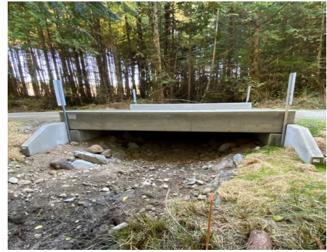
Fish-barrier removal on West Fork Dickey River tributary. Photo: Jeremy Tryall.
