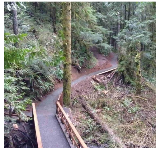
Figure 20: Bridge Improvement Project on the Little River Trail in Clallam County. Photo courtesy of Justin Zarzeczny.
