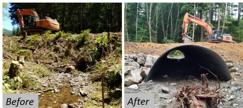
Figure 15: Fish-Barrier Removal on an Unnamed Tributary to Kalaloch Creek. This project replaced a 60-inch corrugated metal pipe (left) with a 16-foot diameter multi-plate culvert (right). A total of 0.7 miles of salmon and trout habitat were opened up as a result of this project. Photos courtesy of Jeremy Tryall.
