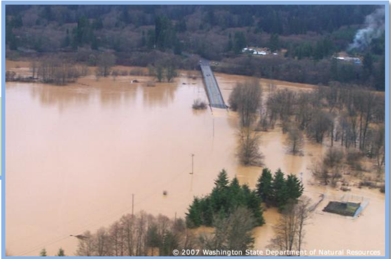
Wind damage that occurred near Raymond and flooding damage between Montesano and Elma from the storm event.
