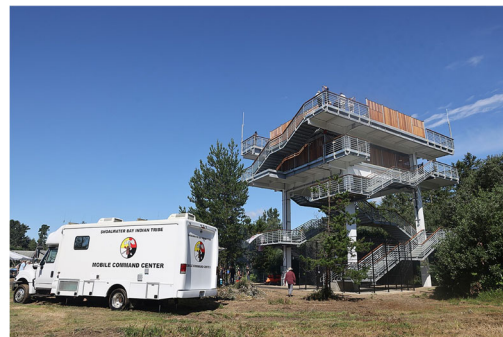
Nation's first tsunami vertical evacuation tower (Washington Military Administrator, 2022).
