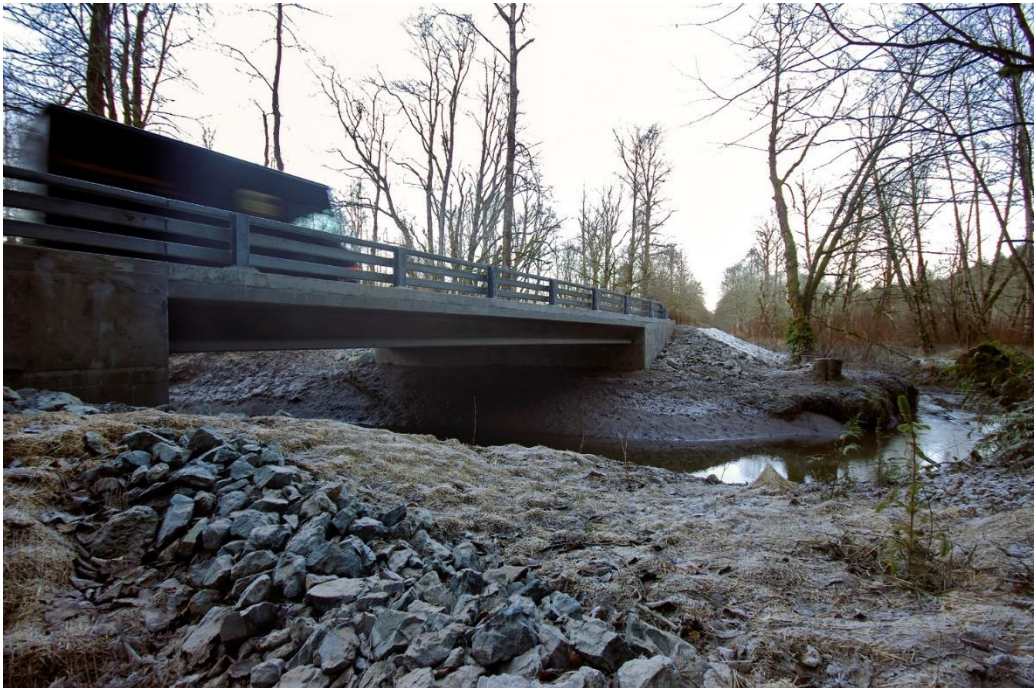
Figure 6-2: Davis Slough Bridge
