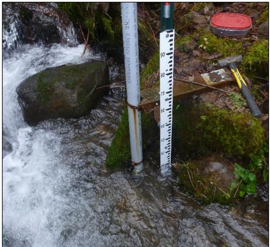
Figure 8-8. Staff gage installed alongside water level sensor housing.
