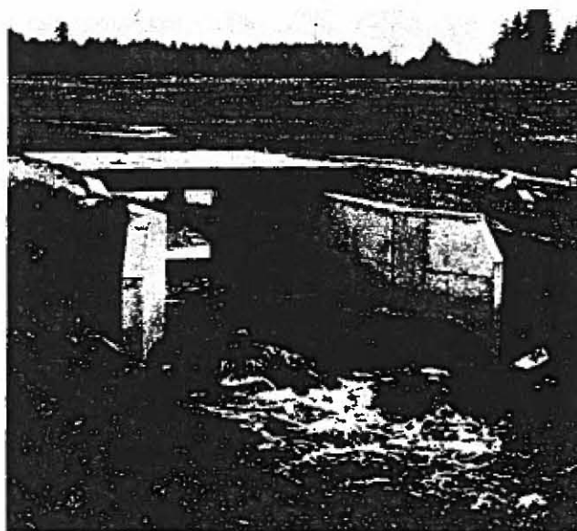
PHOTO 22-21. Fishway on Blooms Ditch diversion dam.
