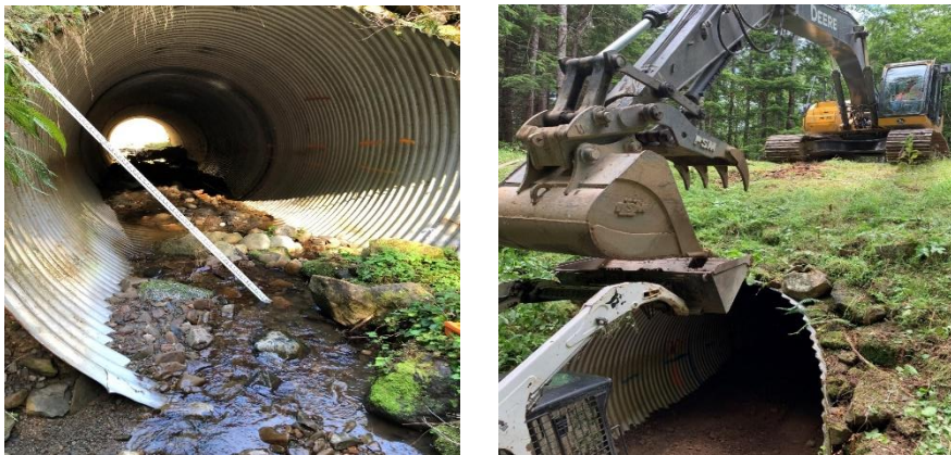
6-2. Culvert maintenance. Photo courtesy of Jeremy Tryall.
