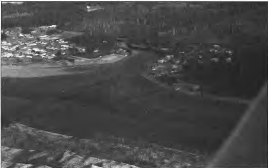
Figure 3. The bridge in the center background at Pacific Beach was damaged by the 1964 tsunami that originated in Alaska. Damage from that event was more common along estuaries than along the open coasts of Oregon and Washington.
