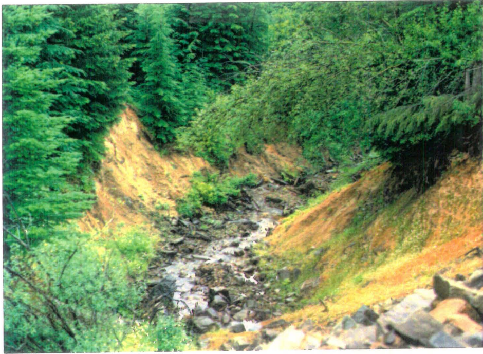
Mineral Creek-Slope Failure due to Upstream Culvert Overtopping
