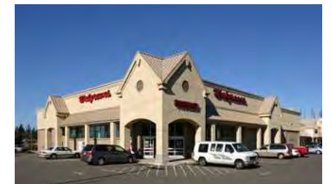
IMAGE SHOWS A 15,000 SQUARE FOOT RETAIL BUILDING LOCATED IN MUKILTEO, WASHINGTON (SNOHOMISH COUNTY), WHICH IS CURRENTLY LEASED TO WALGREENS. SOURCE: CoSTAR
