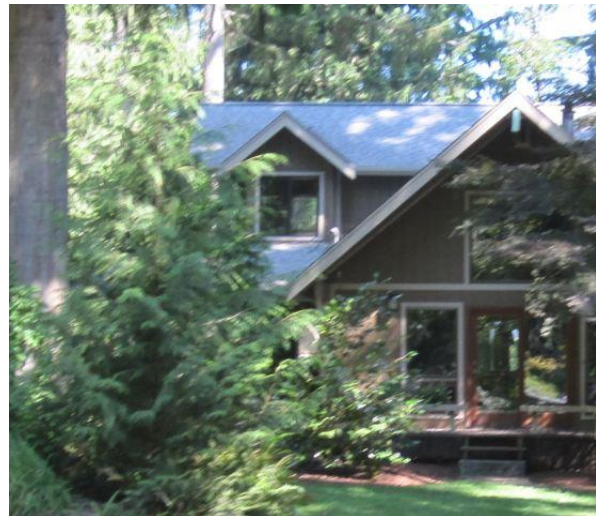
Figure 5-7: Certain types of natural or landscaped plants in close proximity to a home can increase fire risk. Fire resistant plant varieties are a safer choice.
