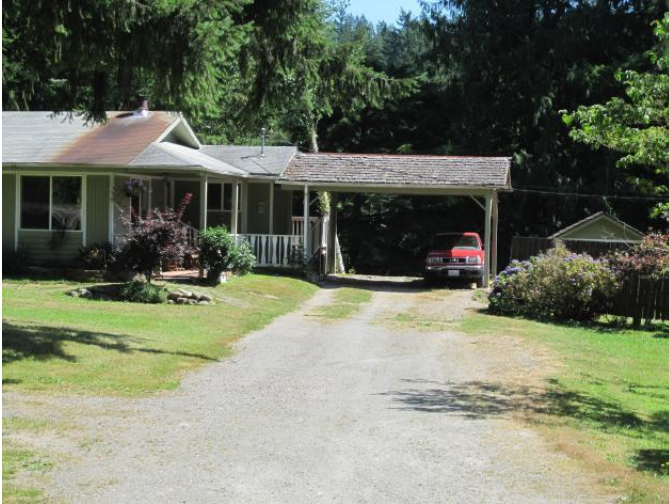
Figure 5-8: Cedar shake roofs are more flammable than composite roofs.
