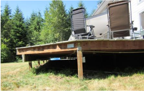
Figures 5-10: Unscreened, raised wooden decks can accumulate flammable material underneath.
