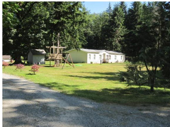
Figure 5-5: Defensible space means using appropriate vegetation around a home to reduce the chances of ignition. You can still maintain a natural setting while reducing fire risk.
