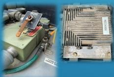
Foam unit is cracked and need to be replaced
