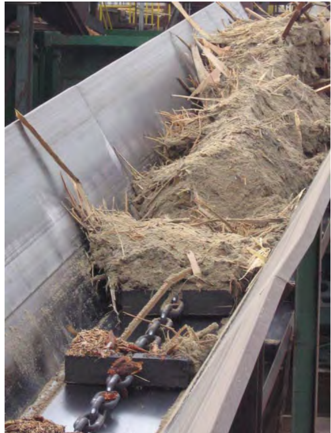
Hog fuel, a by-product of wood product manufacturing, is conveyed to feed Sierra-Pacific's cogeneration facility in Burlington to produce power .
