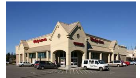
IMAGE SHOWS A 15,000 SQUARE FOOT RETAIL BUILDING LOCATED IN MUKILTEO, WASHINGTON (SNOHOMISH COUNTY), WHICH IS CURRENTLY LEASED TO WALGREENS. SOURCE: CoSTAR
