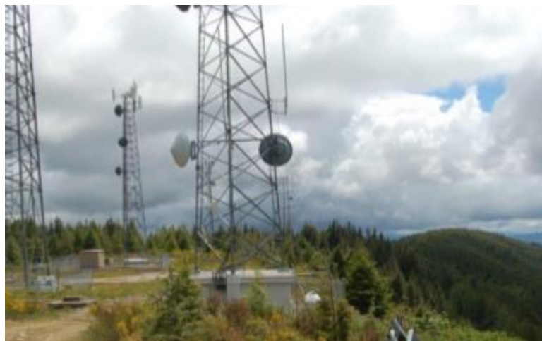
The Radar Ridge Communication Site in Pacific County (South Coast HCP Planning Unit). Photo: DNR
