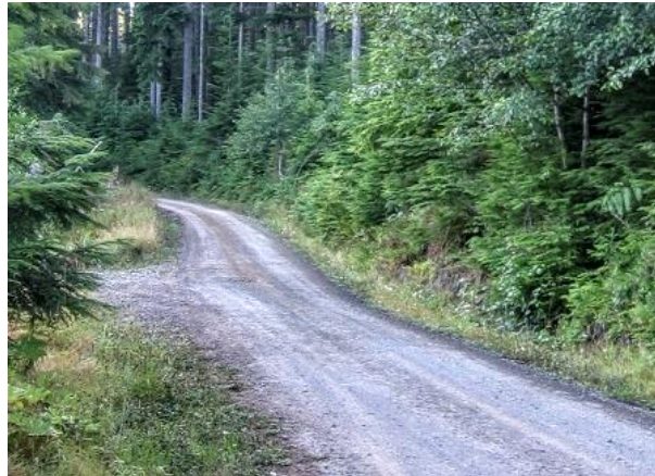
Standard Best Management Practices to Minimize Erosion Include Placing Crushed Surface Rock on Roads. Photo: DNR
