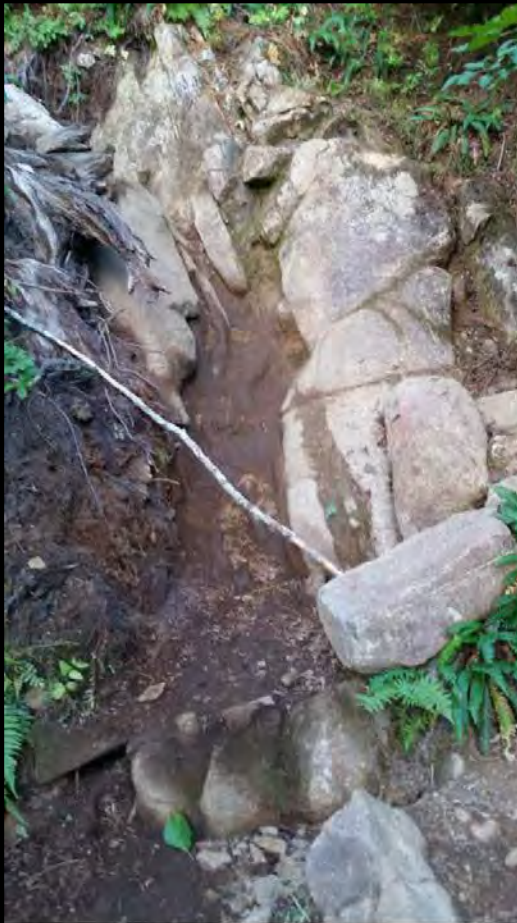
2. Steep Rock at MP 2.67. Serious brushing needed between here and MP 3.16
