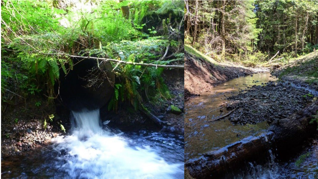
Figure 3. Pictures of the Bear Creek culvert site before and after removal.
