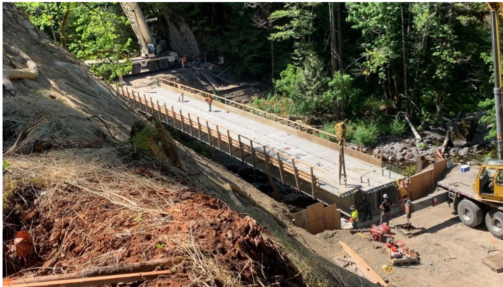
Bridge installation over Steep Creek in Skamania County. Photo: Brett Freeman
