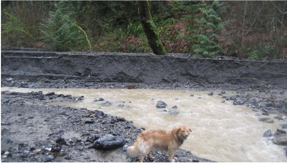
Figure 14 Photograph showing thickness of sediment deposited by debris flood from Tinling Creek. View looking east. Maggie for scale. (Hooks, 2009)
