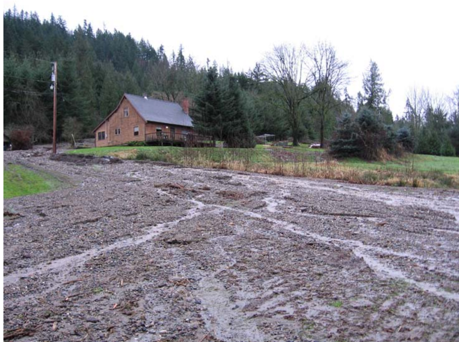
Figure 8. View of debris spread out across lower areas of Site, including driveway and vegetated areas. View looking to the southeast. (Photograph by D. Hooks)
