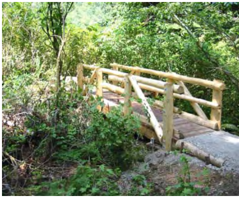
A bridge built on a foot trail to reduce soil erosion and protect a riparian area.
