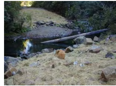
A forested road that was abandoned, with natural drainage restored in the former roadbed.
