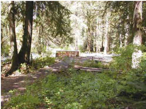
An ADA-compliant platform and trail built at a DNR campground to increase accessibility.
