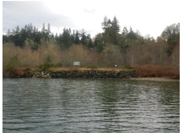
Shoreline armoring along embankment at Floyds Cove
