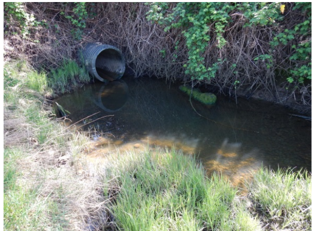
Outlet of Culvert Drain.
