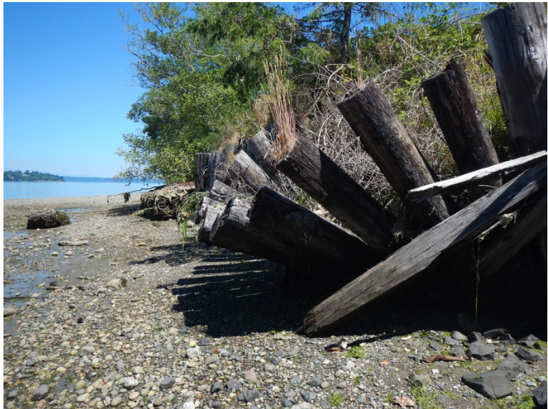
Shoreline armoring along embankment at Floyds Cove
