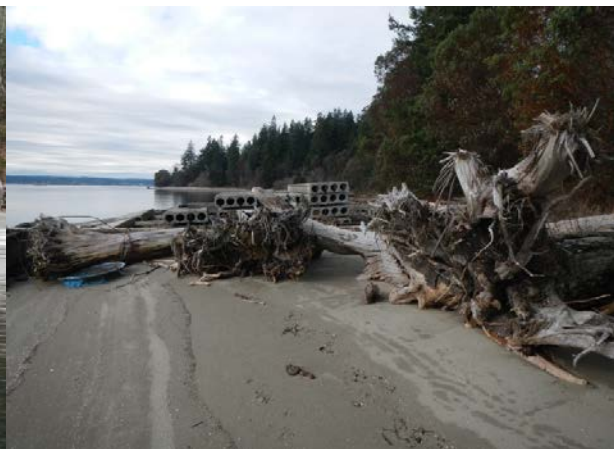
Voided slabs and anchored rootwads at the site
