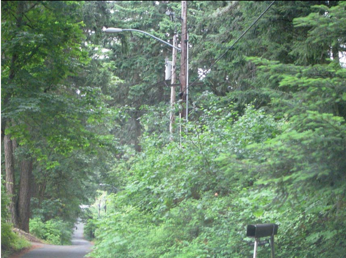
Powerline situated within hazardous fuel situation.
