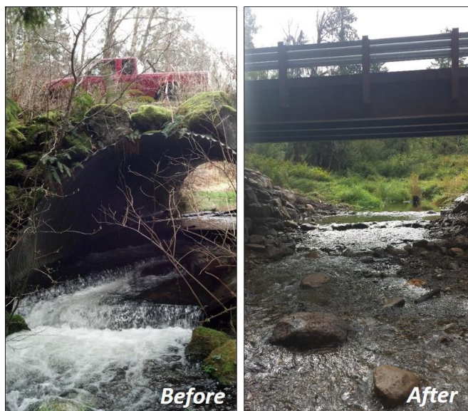
Figure 20: Fish-Barrier Removal on an Unnamed Tributary to the Middle Fork Nooksack River. This project replaced a 142" x 91" pipe arch that was retrofitted with baffles (left) with a 50-foot steel bridge (right). A total of 4.3 miles of salmon and trout habitat were opened up as a result of this project. Photos courtesy of Jason Stuart and Tamra Zylstra.
