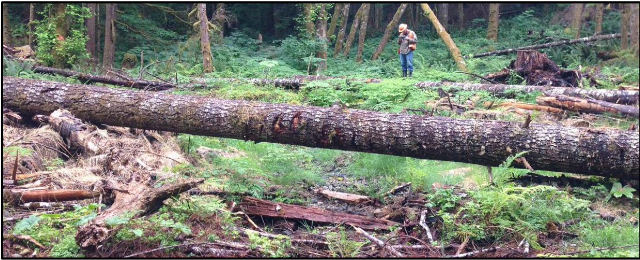
Figure 2. At this crossing, road construction followed by full abandonment resulted in wood placement throughout the RMZ, including within the road prism. This stream had two branches and some stream-associated wetland so DNR staff elected to place longer logs across the entire feature instead of individual pieces for each crossing.
