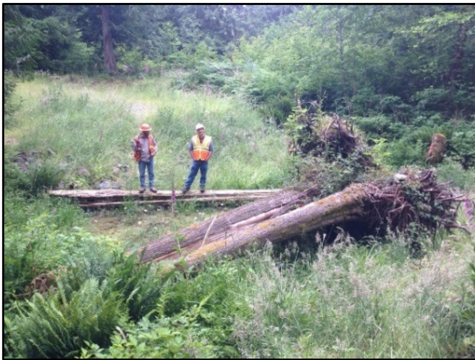
Figure 7. Wood placement within a decommissioned road crossing may result in disturbance to the channel when the road is reopened, but this placement also deters off-road vehicle access which can be a more severe and persistent disturbance agent.
