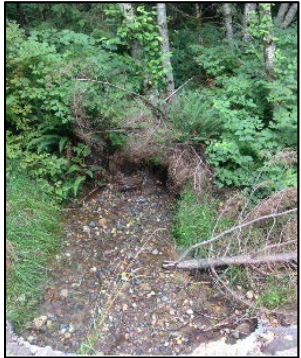
Figure 5. While the RFRS doesn’t prescribe a minimum diameter for wood requiring placement into or adjacent to the stream, DNR staff should use professional judgement as to whether wood placement is stable (i.e., has little risk of moving down stream during high flows) and functional. At this crossing associated with road reconstruction, conifer saplings are placed along the edge of the stream for erosion control in addition to meeting apparent RFRS requirements.
